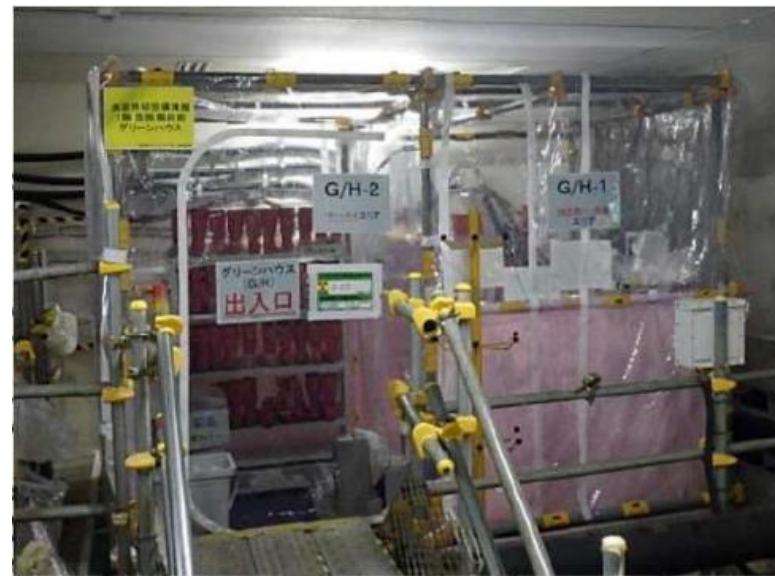
Figure 18 Equipment exchange after the change
