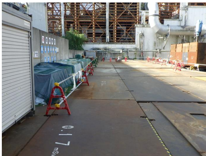
Figure 9 Shielding with crushed stone and steel plates
