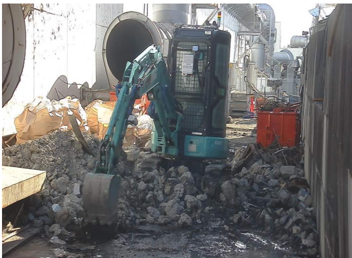
Figure 11 Unmanned heavy machinery removes high-dose debris
