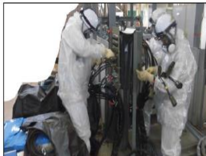
Figure 14 Mock-up status (cable connection and disconnection)
