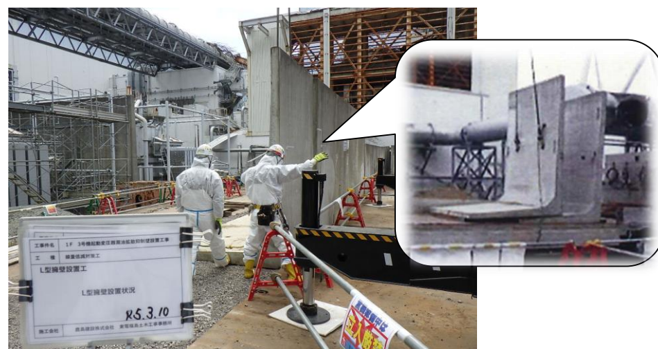
Figure 10 L-shaped retaining wall
