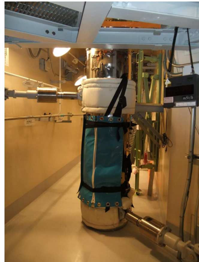
Temporary radiation shielding with tungsten mats(e.g.) 21
