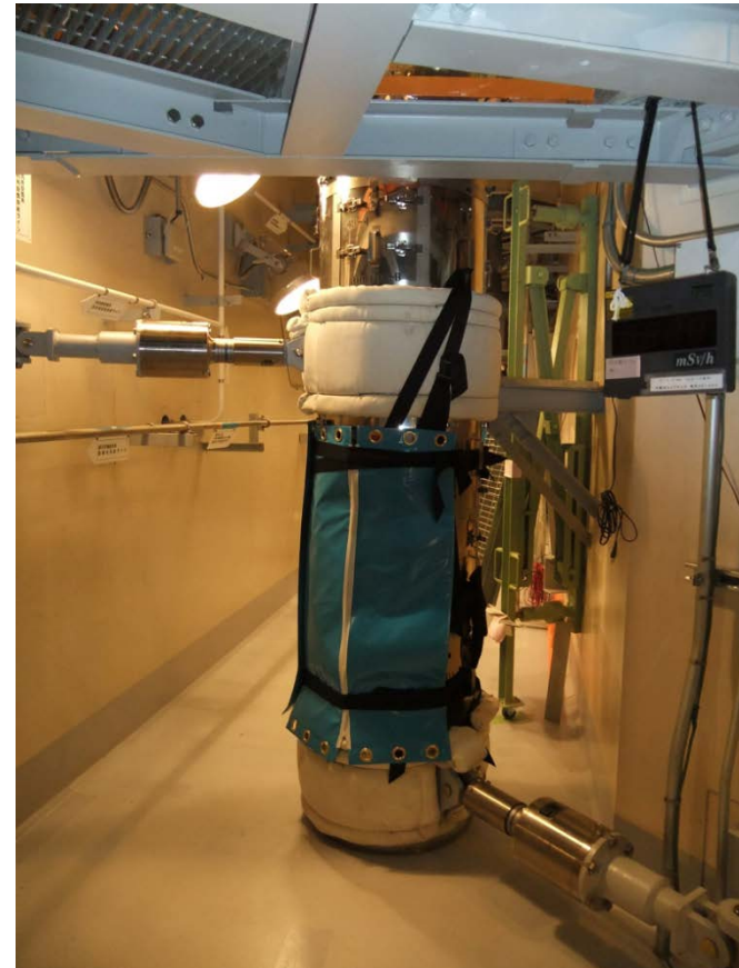
Temporary shield using tungsten mats (Example)
