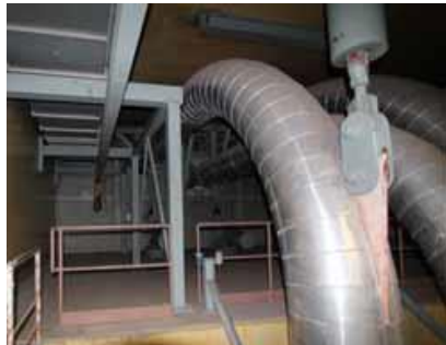
Main steam piping (in the case of Unit 2)
