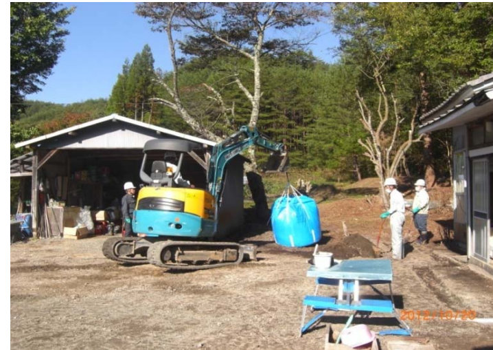
4) Stripping work of the topsoil
