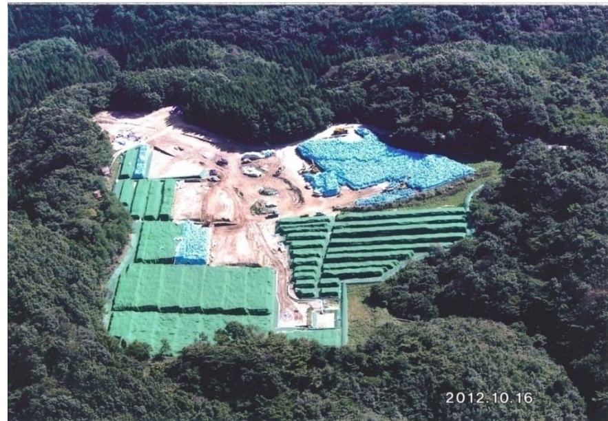
3) Panoramic view of the temporary storage yard
