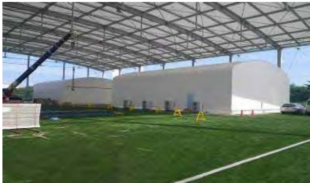
WBC center at Hirono Football Stadium
