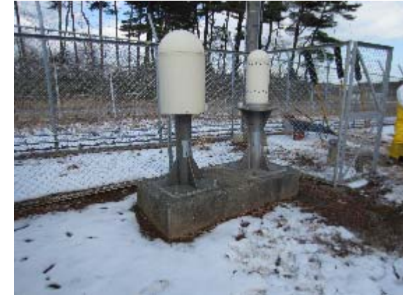
Monitoring post No.2
