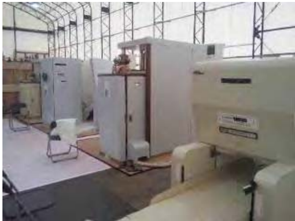
Inside the building
