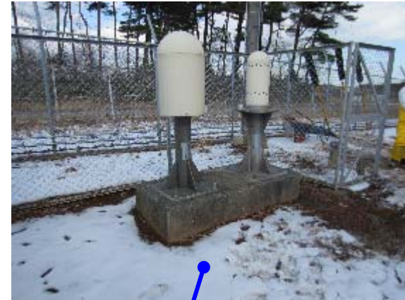
Monitoring post No.2
