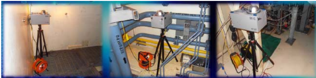
Reactor Building RMVS
